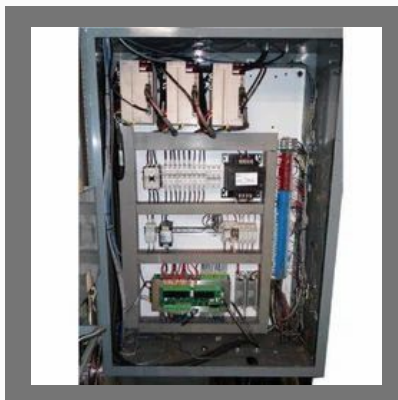
Electric Control Panel Installation Service
